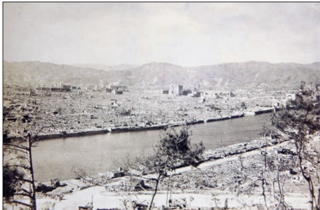
A river winds its way through the devastation.
