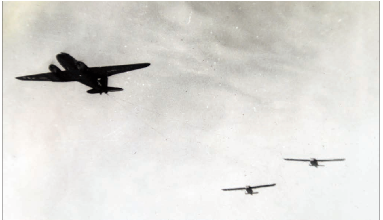
A C-47 tows two gliders during the war. Both the transport pilot and the glider pilot could release the tow rope if need be. The glider pilots only took over total control of the aircraft with about two minutes left in the mission. On D-Day, they had to land with no lights or landmarks.
