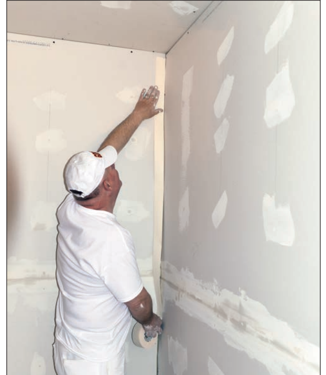
Department Adjutant Randy Tesdahl measures out some tape in one of the interior spaces at Legionville's new education center. If you would like to volunteer, contact Camp Director Roy Kruger at 218-829-3094.
