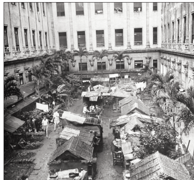
Shacks were constructed in the courtyard of the main building at St. Tomas. (U.S. Army photo)
