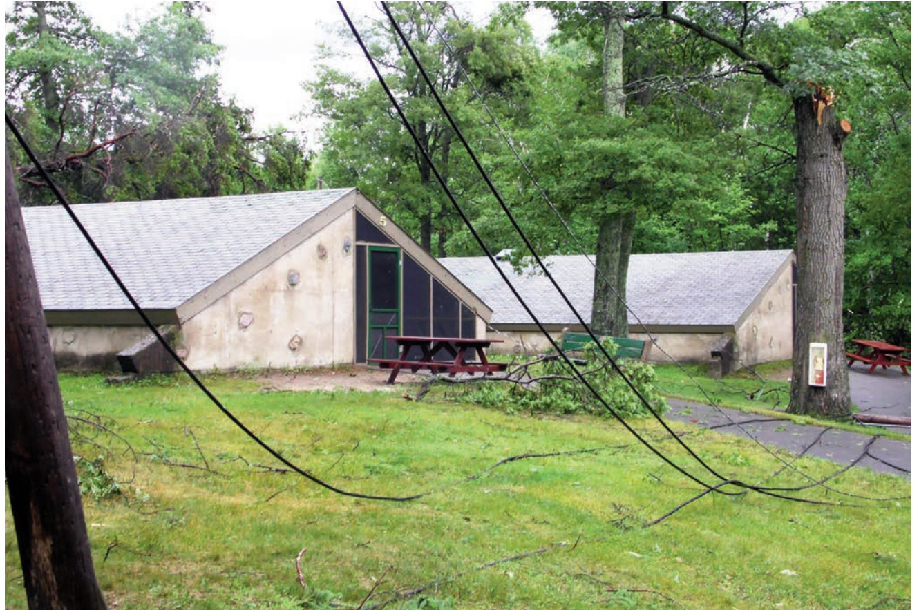
Downed power lines lay on the ground near Cabin 5. The power was immediately cut after the storm so the wires were not live.
