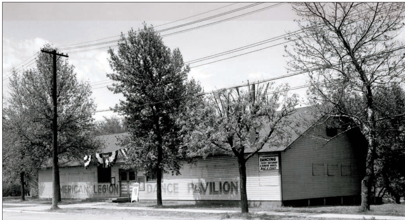
FIRST PLACE, $300 WINNER -- The American Legion Dance Pavilion was built by Breckenridge Post 53 with $6,000 donated by members. It included a 100 by 50 foot maple dance floor along with a band shell, concessions, restrooms, a checkroom and rotary fans. It opened on June 19, 1929, to 1,400 dancers. Bands that played at the Pavilion included Glenn Miller, Harry James, Tommy Dorsey and Lawrence Welk. Other artists that played there included Conway Twitty, Bobby Vee, and Jerry Lee Lewis. It was torn down in the 1980s. Submitted by Tom Matejka.
