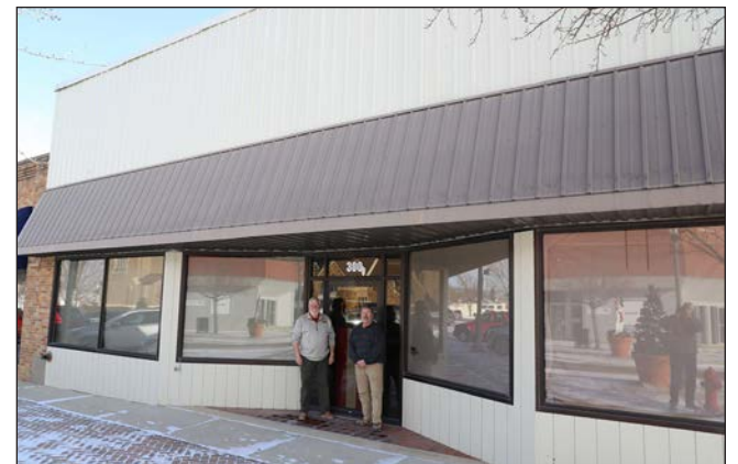
This nondescript building will have windows decorated with American Legion emblems as American flags. It doesn't look like a post, but it will by the end of March.
