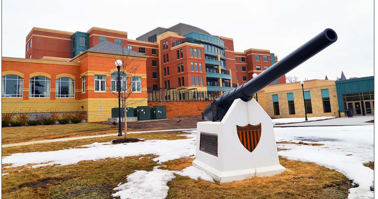
Building 22 was dedicated in March. It will have 100 private rooms and many amenities. A Spanish-American War cannon sits on the lawn outside the new Veterans Home in Minneapolis.
