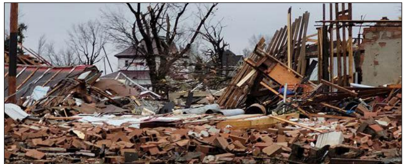
Buildings in Taopi were flattened by a tornado on April 12.
