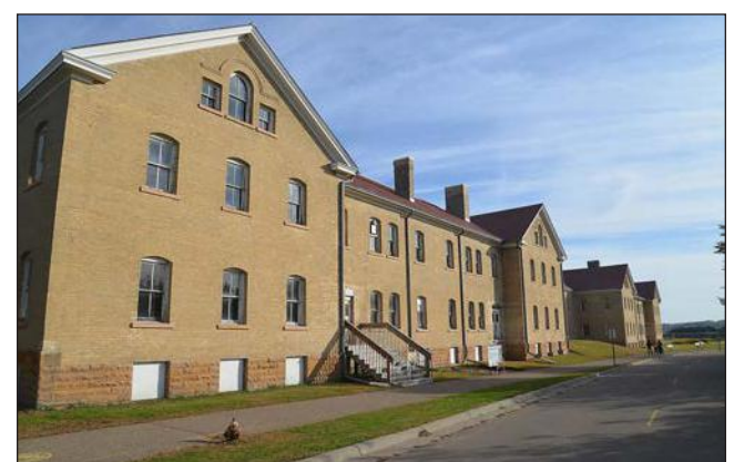
NEW VISITOR CENTER — These cavalry buildings, built in 1904, along with a nearby ordnance warehouse from the 1870s, will host the new visitor center once a capital campaign is finished.
