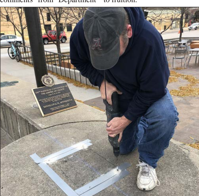
A Twin City Monument employee saws into concrete on Nov. 9 at the spot of new plaque at Peavey Plaza.
